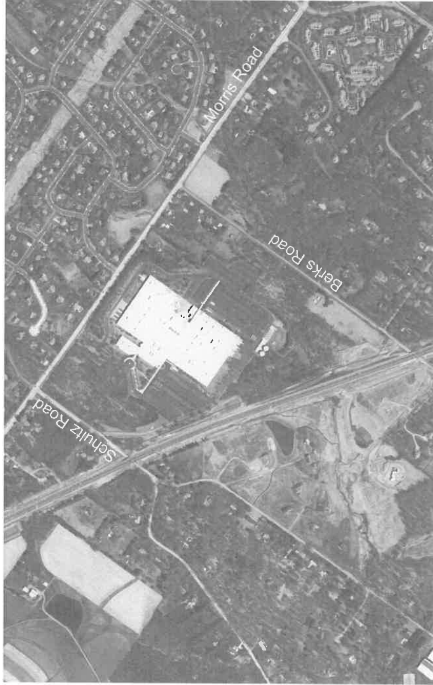
2750 Morris Road - Building "D" South MCPC #19-0007-001
