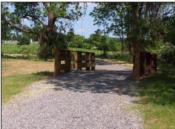
A view of the entrance to the new Zacharias Trail, from the access point on Green Hill Road.
