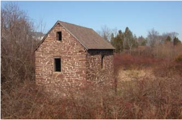
The Smith pioneer house was acquired by the Township.
