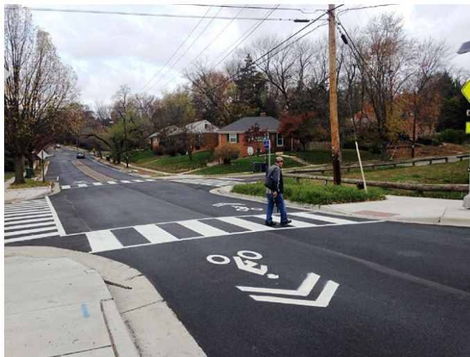
Curb bumpout with Shortened Pedestrian Crossing Distance Source: Hillary Orr via FHWA.
