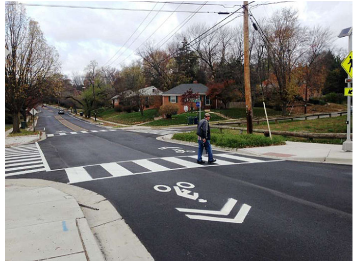
Curb bumpout with Shortened Pedestrian Crossing Distance Source: Hillary Orr via FHWA.
