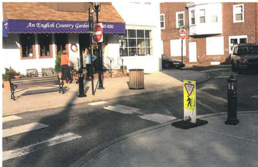
Bumpouts in Jenkintown were used to narrow West Avenue, making it easy for pedestrians to cross from one side to the other.
