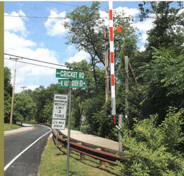
This red and white floodgate can be lowered when the road floods to stop vehicles from driving into unsafe floodwaters.
