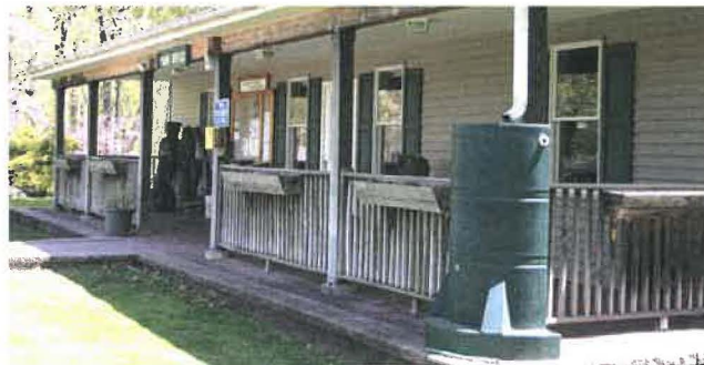
This rain barrel at Green Lane Park helps with the county's MS4 stormwater permit requirements.
