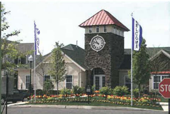
Station Square is a suburban mixed use development next to the Pennbrook Station in Lansdale.
