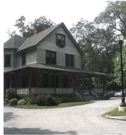
This historic home in Ambler has been reused as an architect's office.
