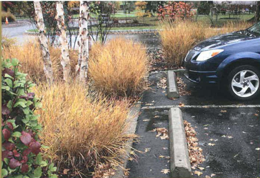
Bioswales and porous paving allow water to infiltrate into the ground and help with groundwater recharge.
