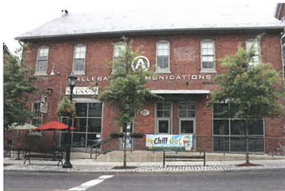
Reuse of historic buildings is the best way to preserve town character.
