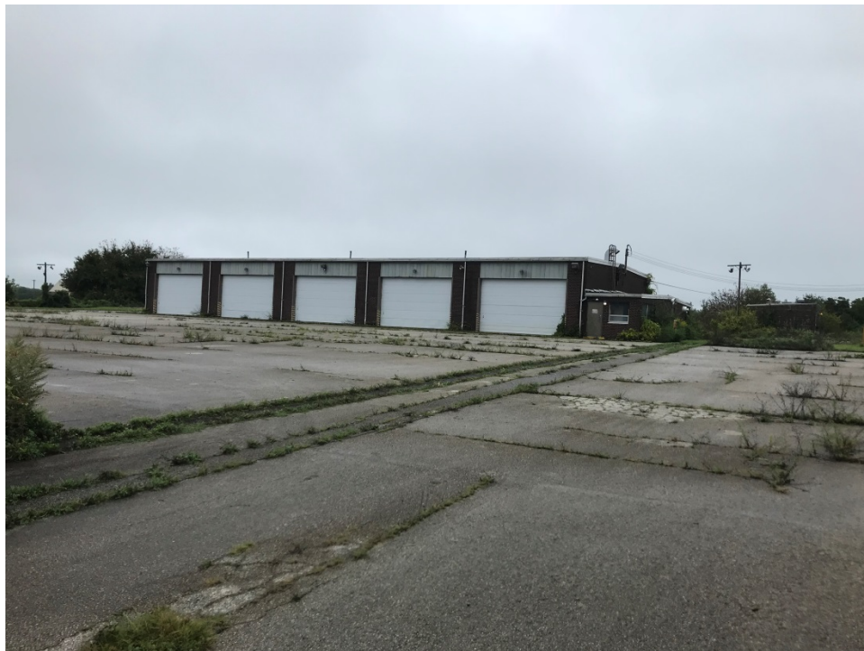
Photograph 12. OMS Building and MEP Parking Area
