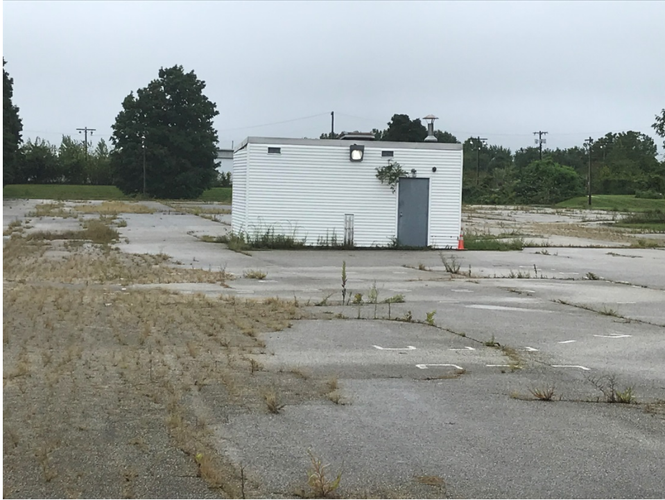
Photograph 5. Potable Water Pumphouse
