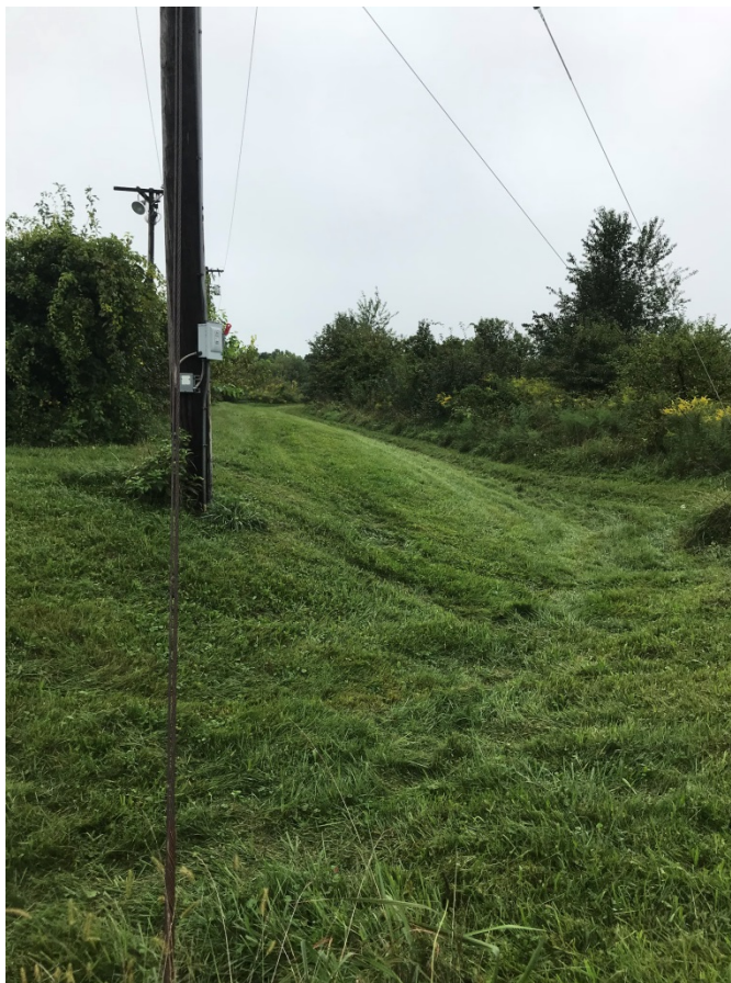
Photograph 10. Swale North of the OMS Building (Facing North)
