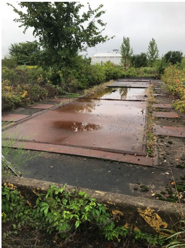
Photograph 16. Nike Missile Silo Lift
