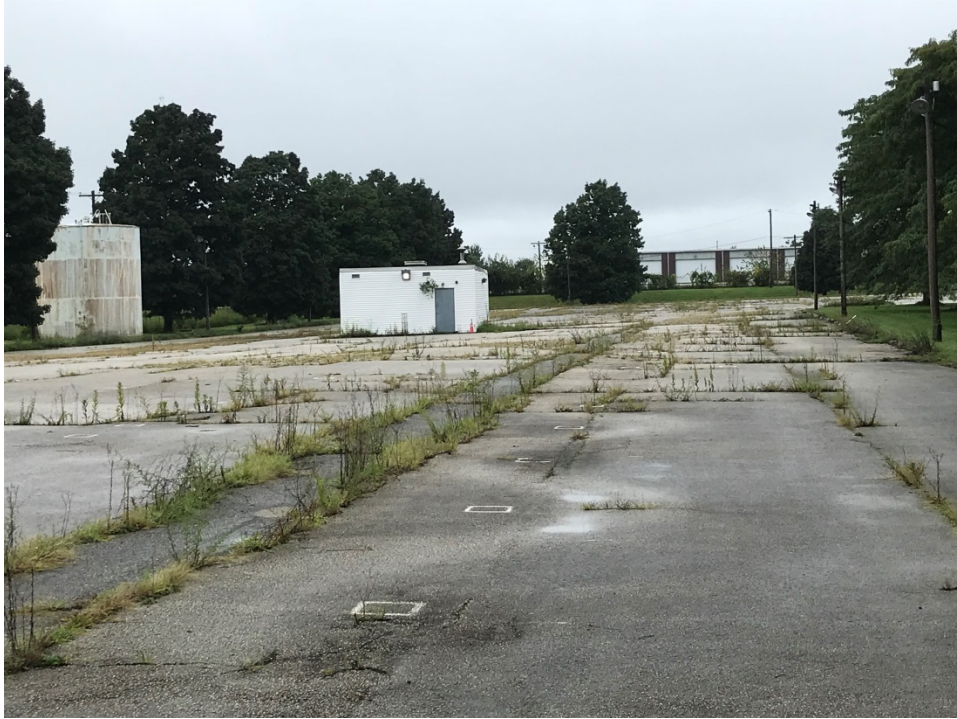
Photograph 23. View of North Penn USARC (Facing North) with Potable Well Pumphouse, OMS Building, and AST
