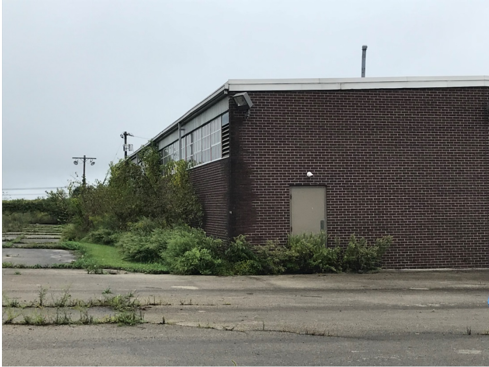
Photograph 21. Rear Side of the OMS Building
