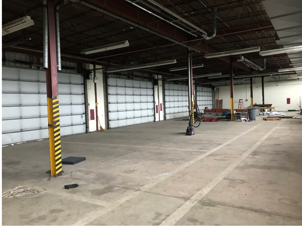
Photograph 13. Interior of OMS Building
