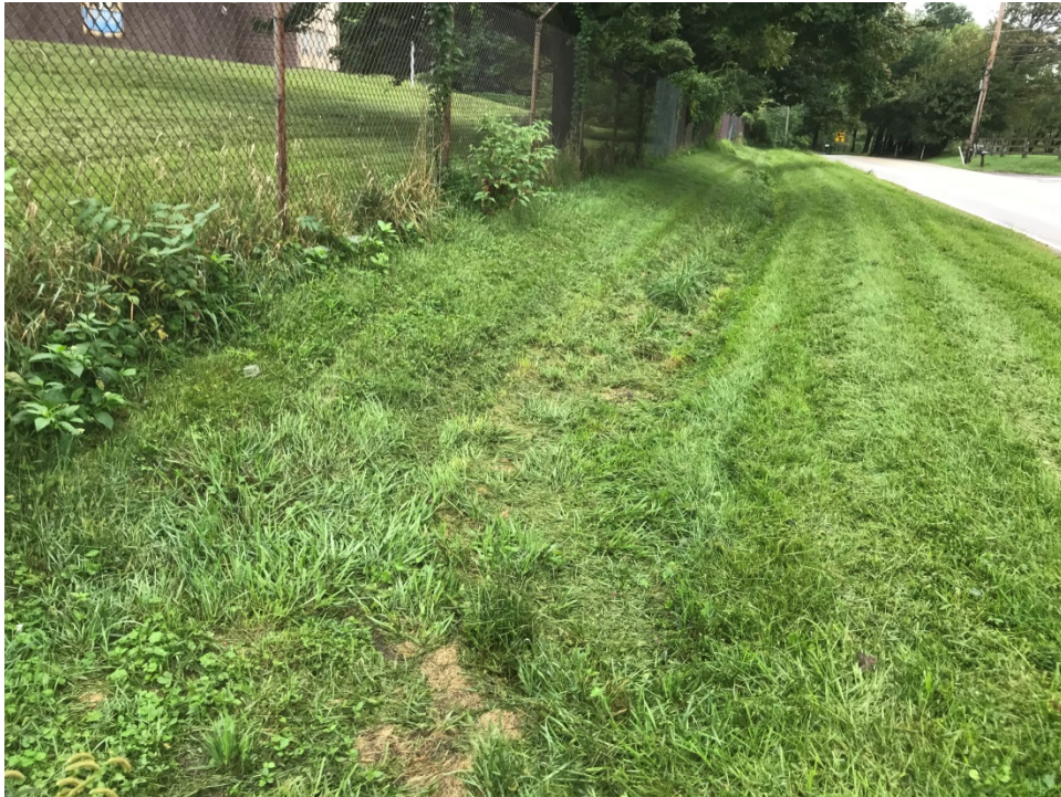
Photograph 4. Ditch Outside the Property Fenceline, Parallel to Berks Road
