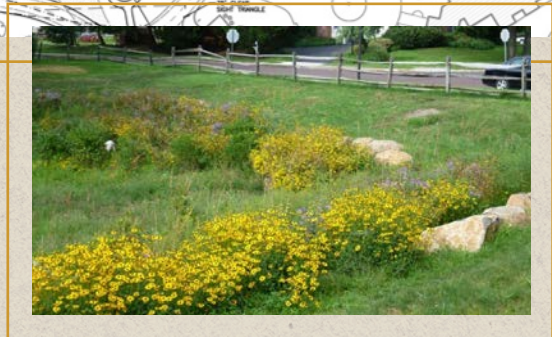
A landscaped forebay
