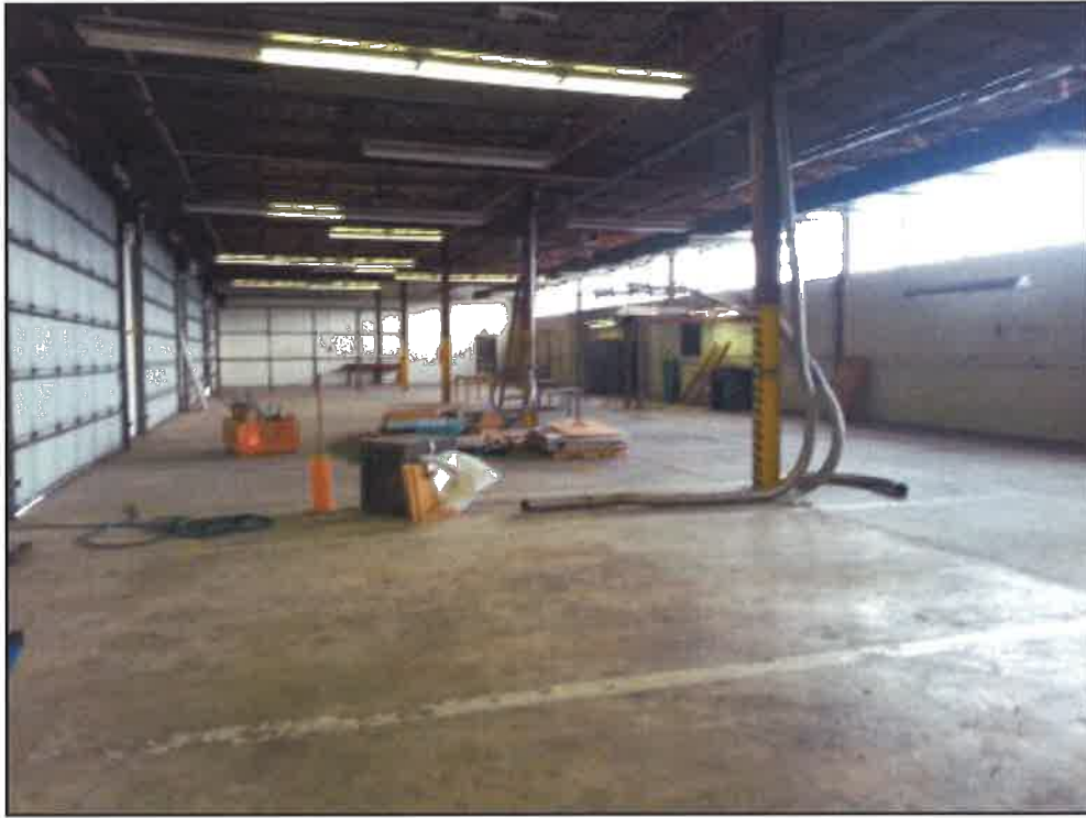
Photograph 23: Inside of OMS building. No evidence of service pits.
