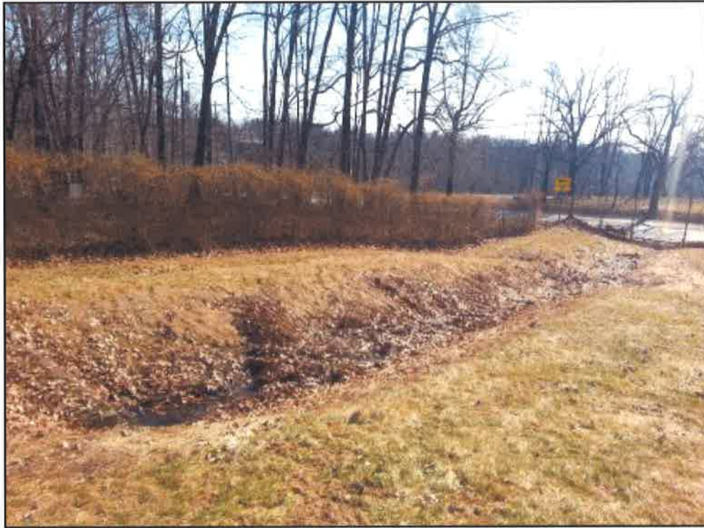
Photograph 25: Drainage Ditch (AOC G).
