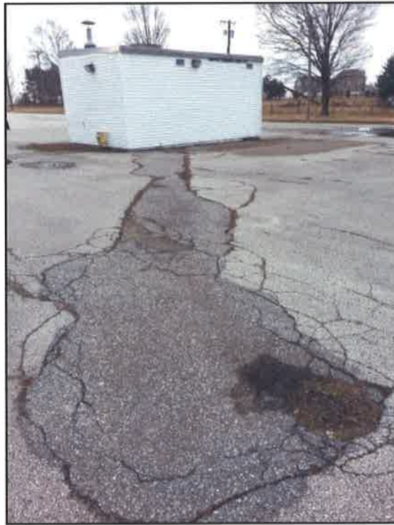
Photograph 19: Newer potable well flush with parking lot in foreground with the potable well house in the background.
