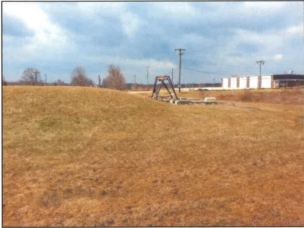
Photograph 35: View of sand mound from side with OMS building in background.
