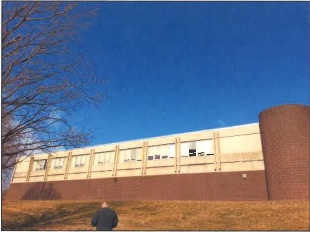
Photograph 1: Front of administration building.
