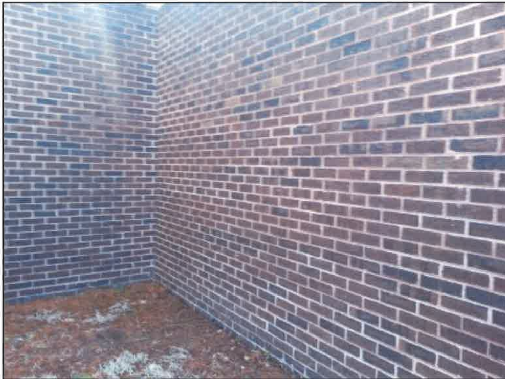
Photograph 14: Assumed location of former remote fill for the former 20,000 gallon heating oil UST.
