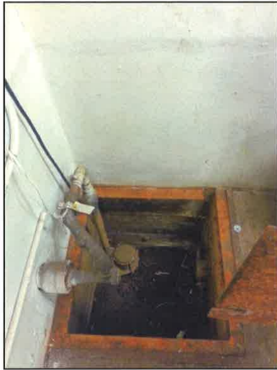
Photograph 13: Sump observed in boiler room of administration building.
