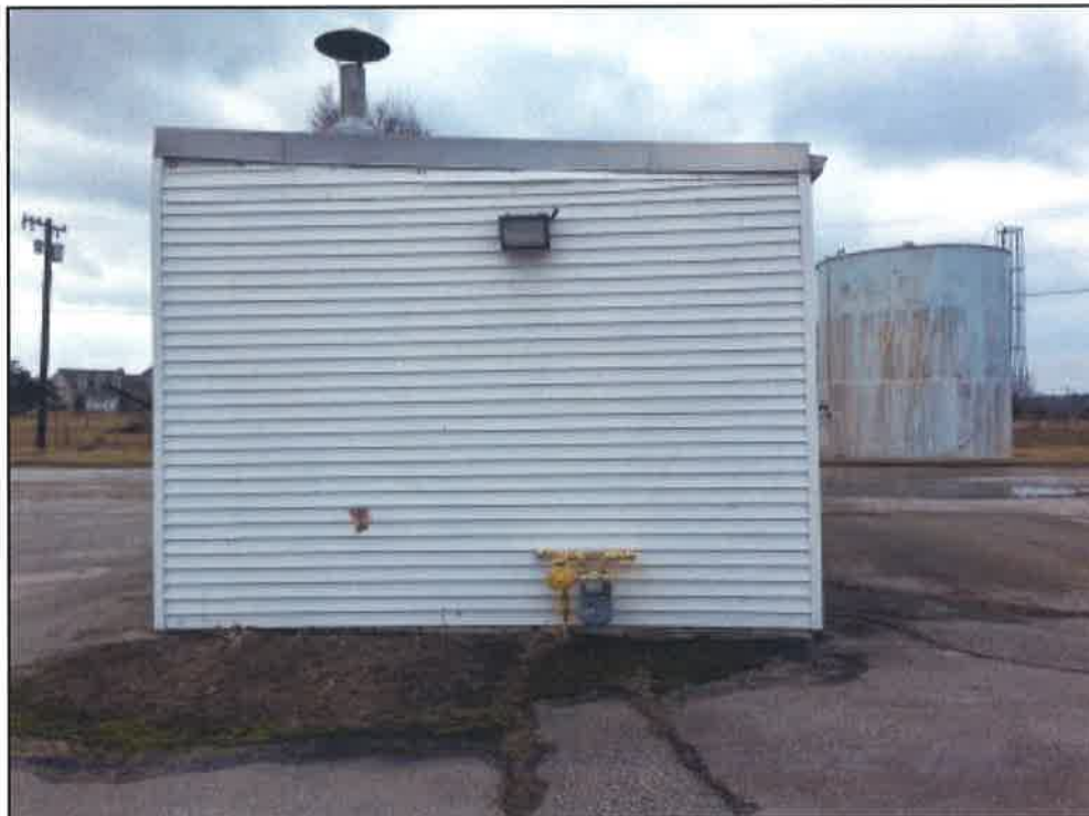
Photograph 18: Potable well house and location of former heating oil AST and spill location.
