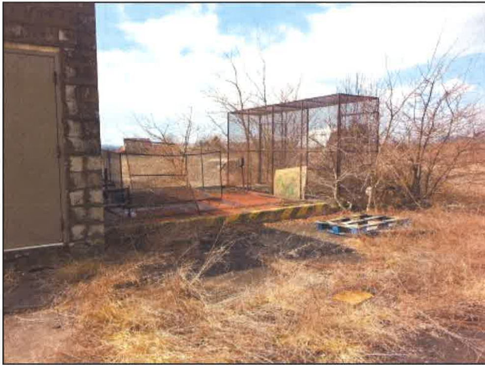
Photograph 33: Area behind fire protection pump house.
