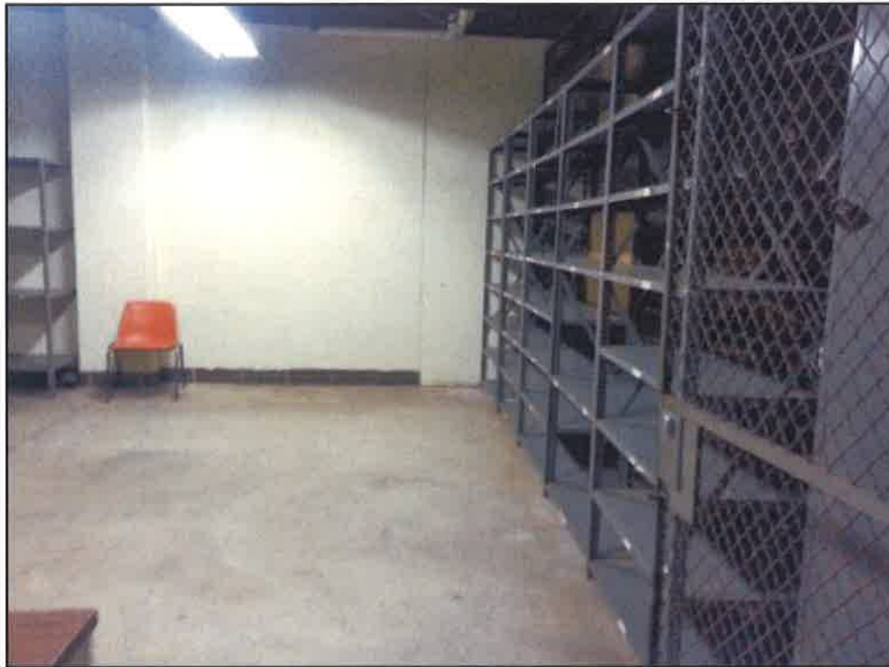
Photograph 3: One of multiple storage areas located on the first floor of administration building.
