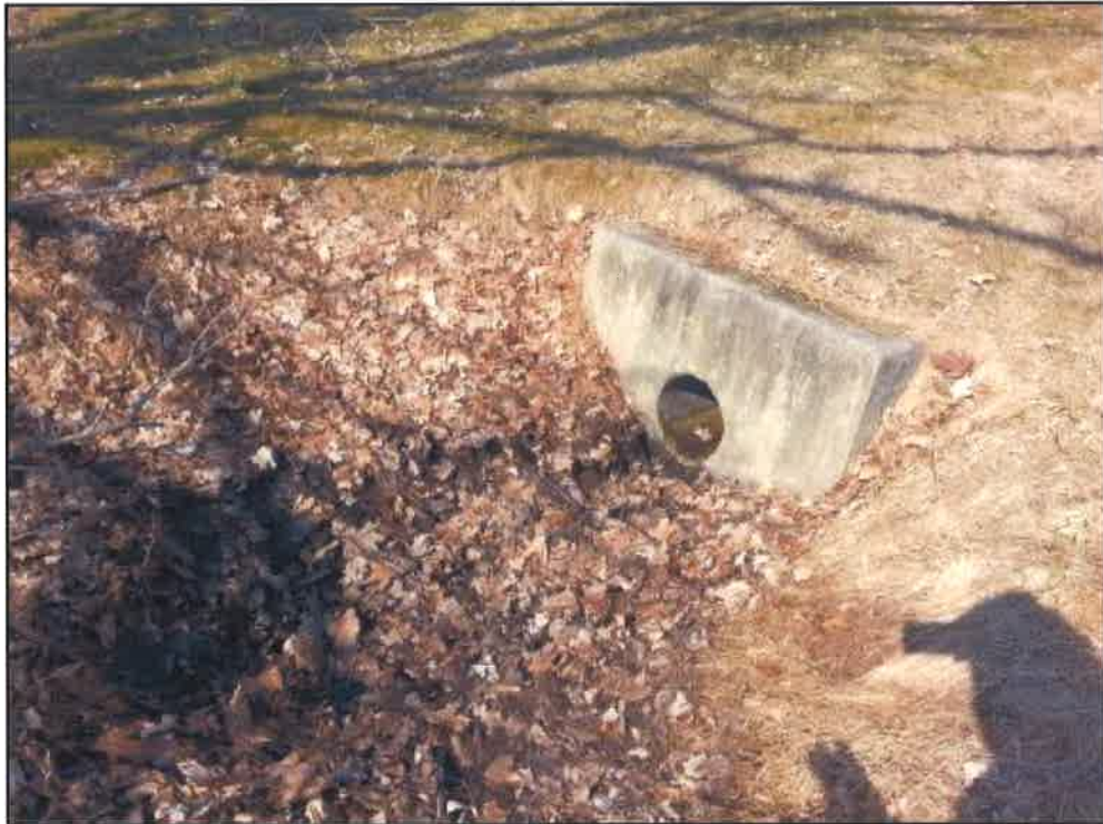
Photograph 36: Drainage ditch (AOC T).
