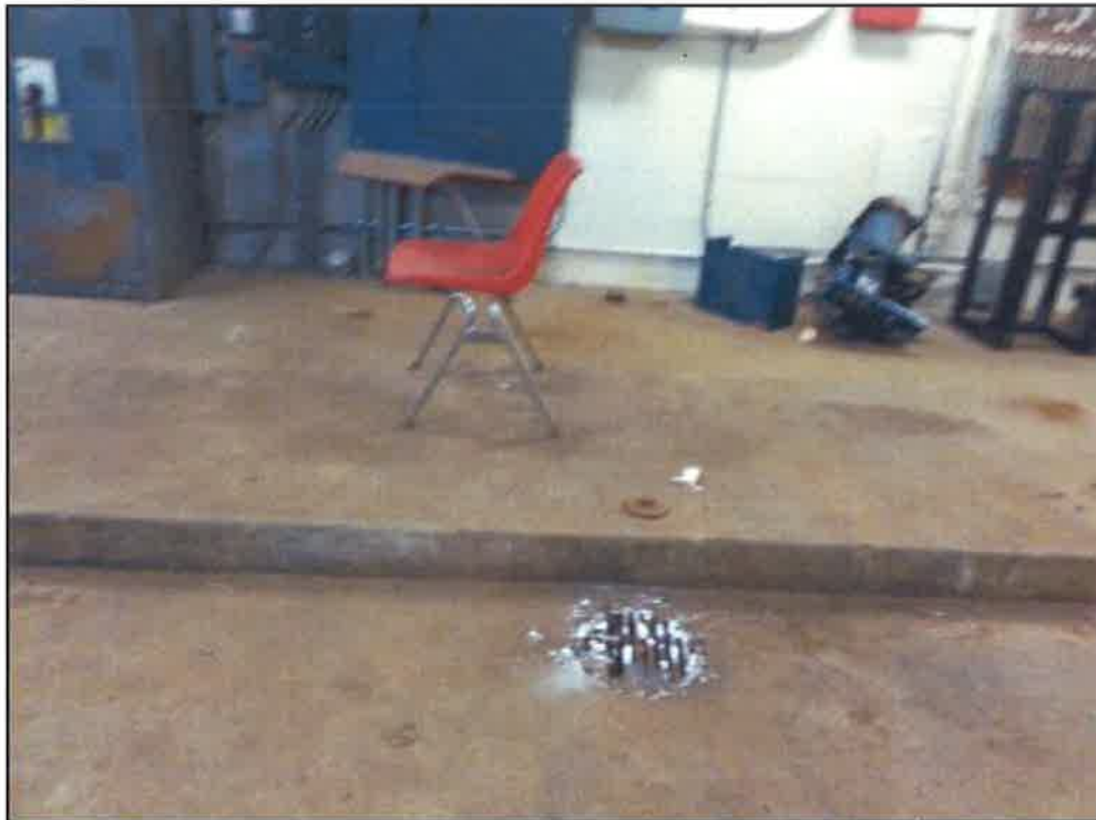
Photograph 12: Floor drain observed in boiler room of administration building.
