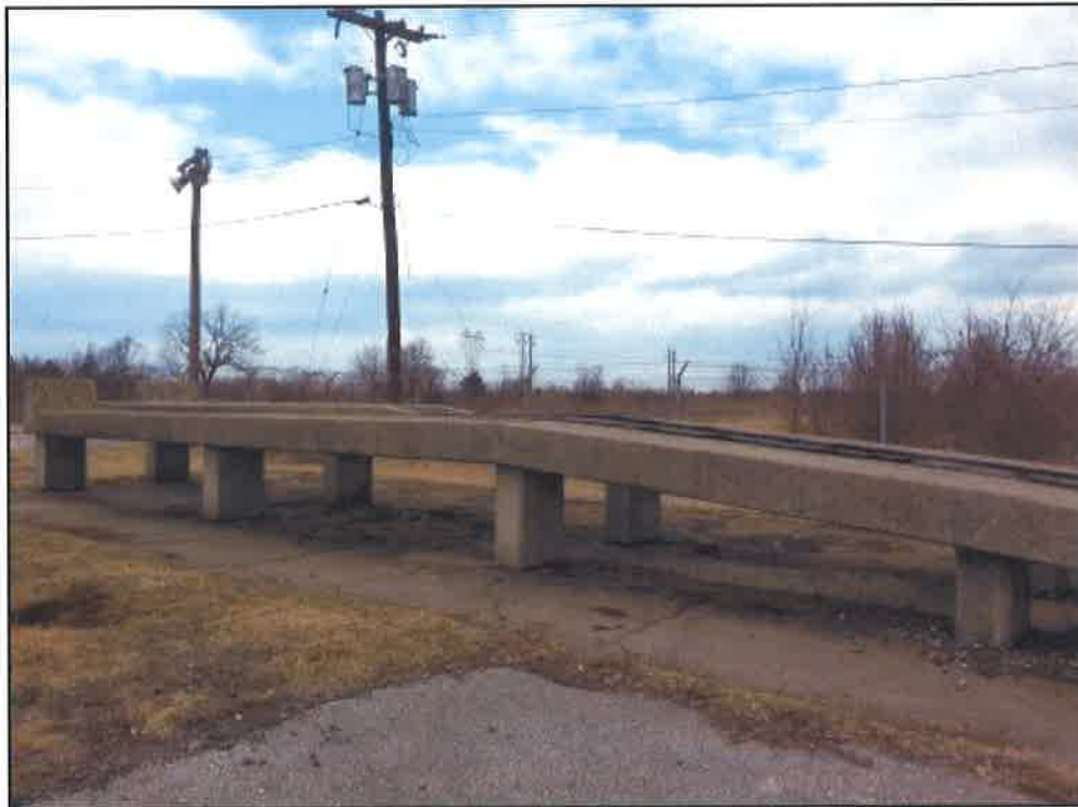
Photograph 22: Grease rack located adjacent to the OMS building.
