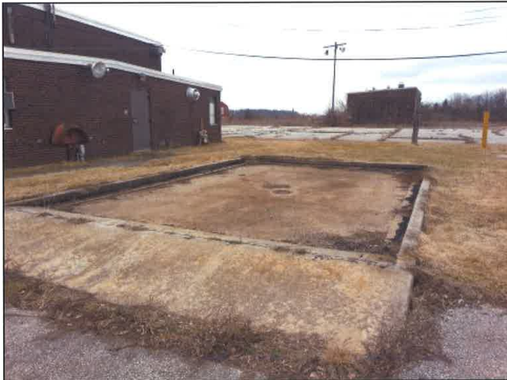
Photograph 20: Wash rack located adjacent to the OMS building.
