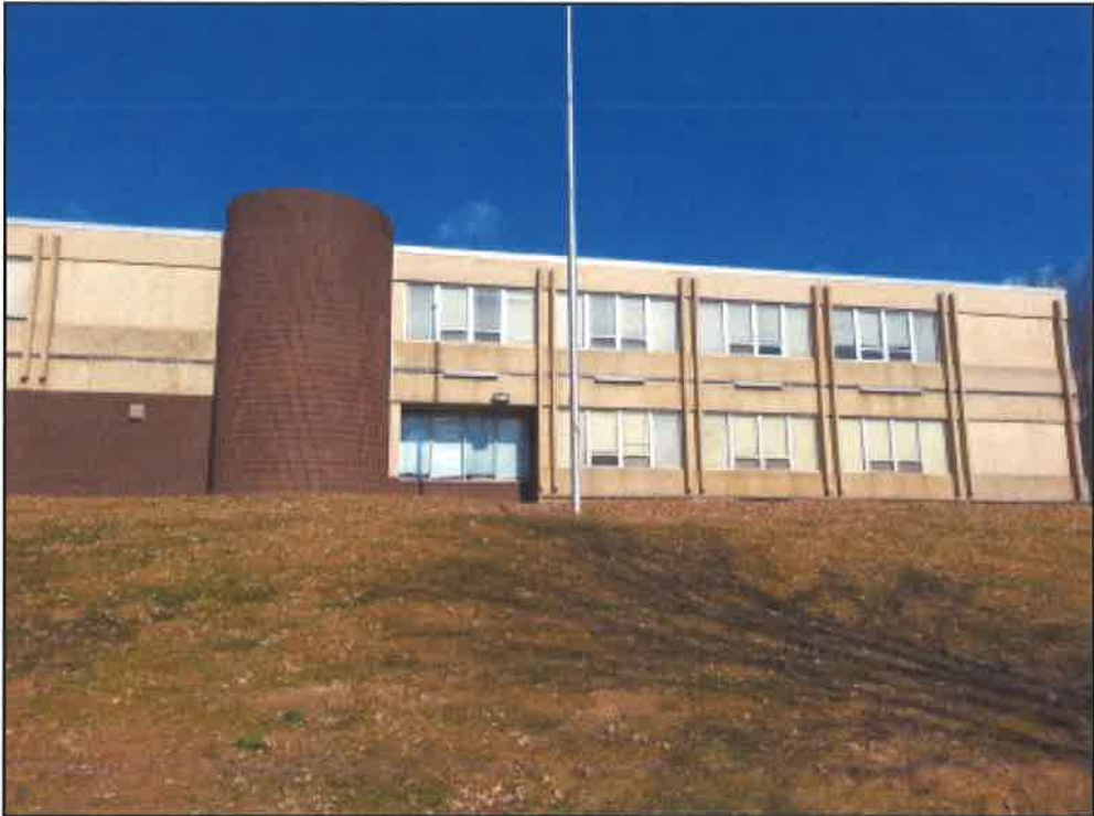
Photograph 2: Front of administration building.
