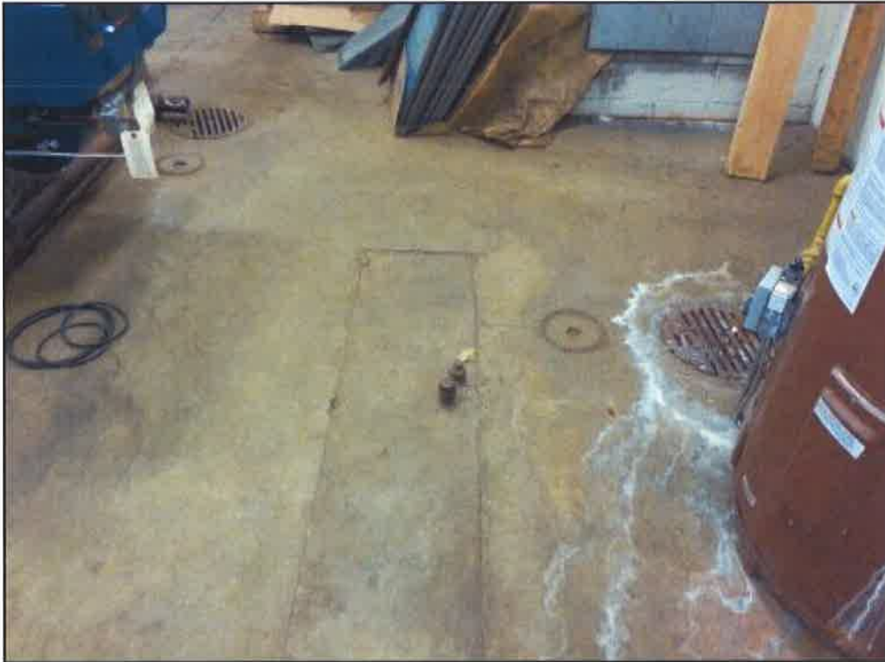
Photograph 8: Former 20,000 gallon pipes cut off above floor grade.
