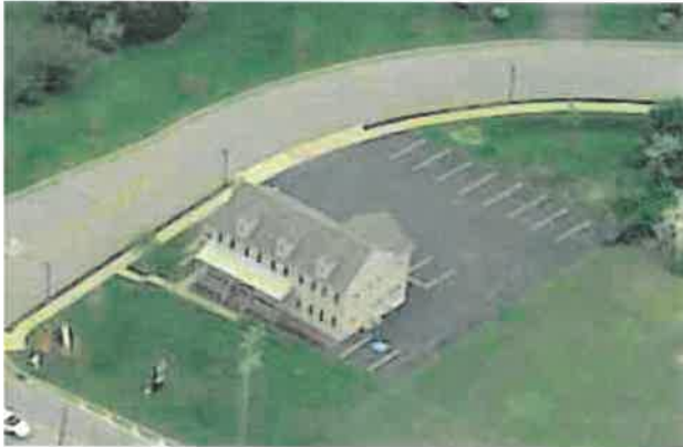
Offices at Germantown Pike and Heritage Drive in Worcester.
