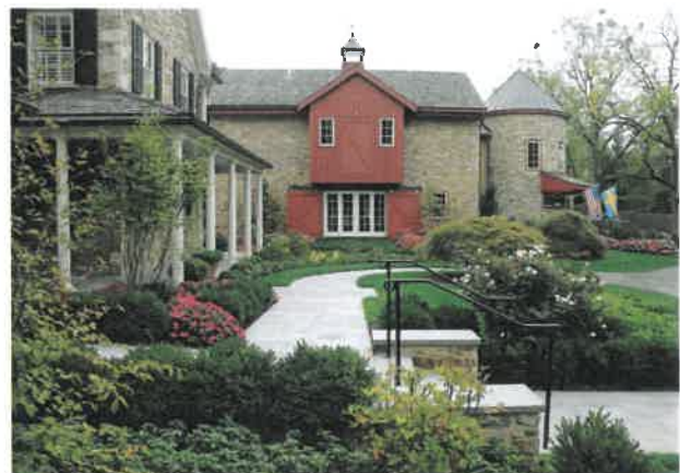
Meitner Family Property, Whitpain Township, PA: this historic rural farmstead was converted and expanded into offices and new residences.
