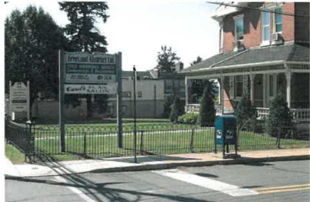
Collegeville, PA: an older home with historic character has been converted to office and other business uses.
