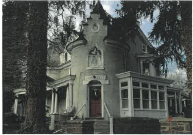
Worcester: a prominent older home on a major thoroughfare.
