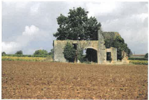
There are many alternatives to demolition of historic resources. Sometimes people just need some time to get the facts and understand options.
