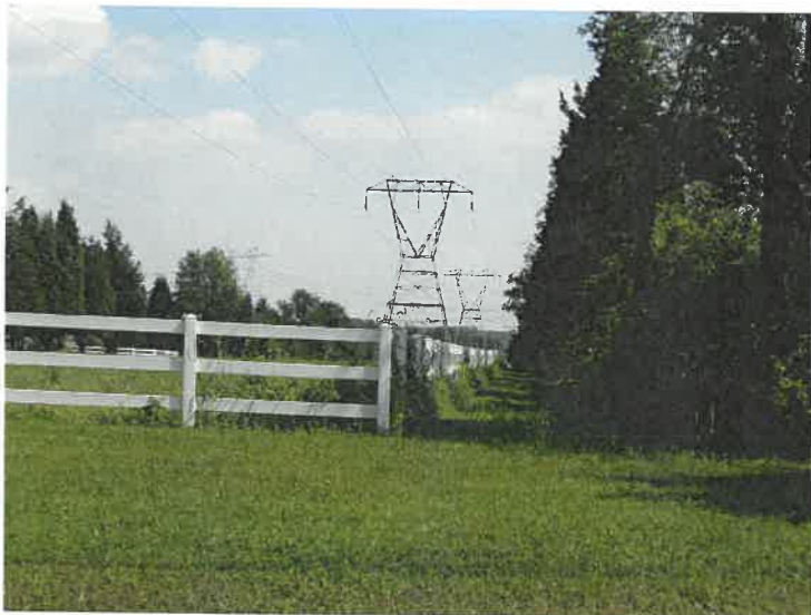
PECO ROW at Wentz Church Road.
