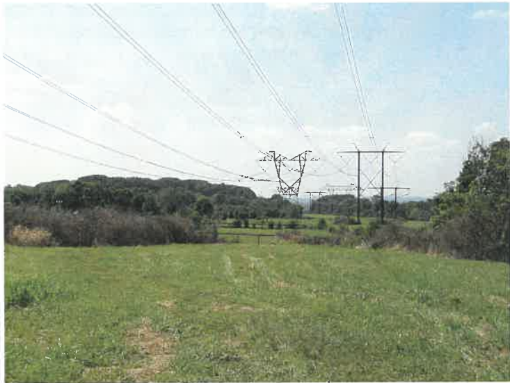
PECO ROW at Berks Road.
